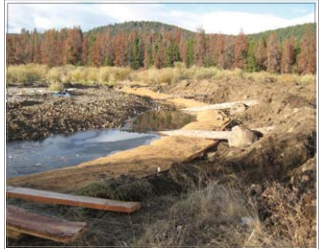
Bank Stabilization -Log vanes, constant radius curve and willows plantings
