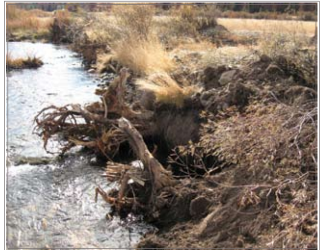
Rootwad bank stabilization
